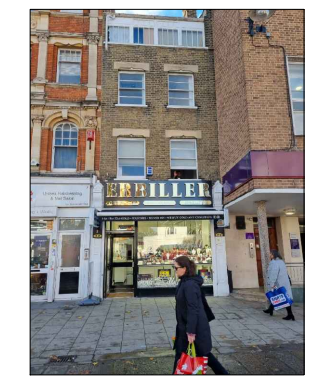
4 FASCIA SIGN PICTURE AFTER WINDOW CANOPIES AND VERTICAL SIGN HAVE BEEN REMOVED
